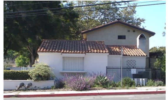
Braemar Sewer Lift Station
